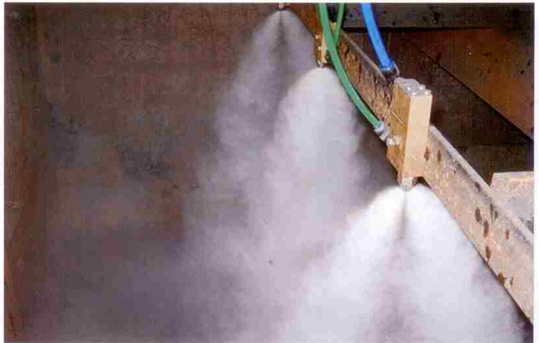
Dry Fog Nozzles Placement for Transfer point.
